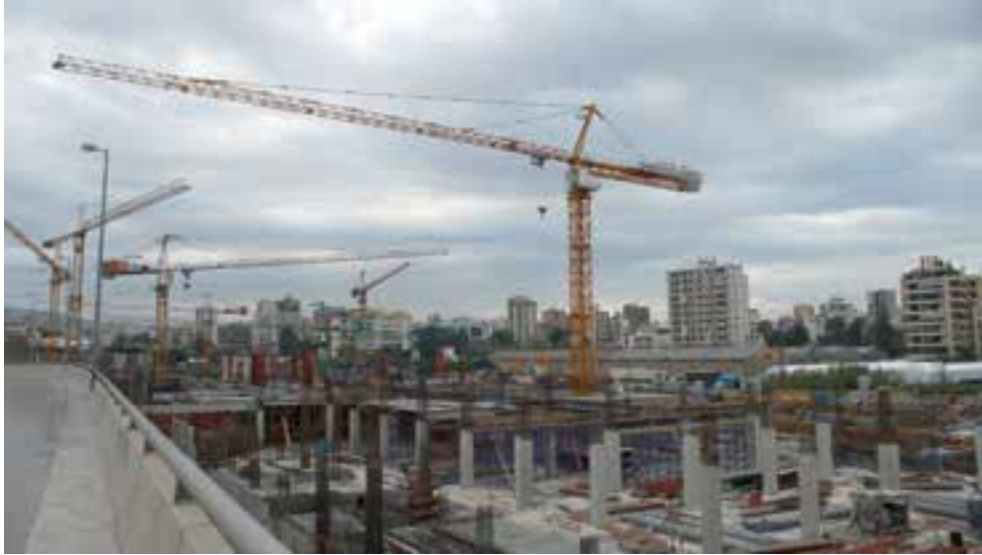
Construction site, Beirut, 2012
